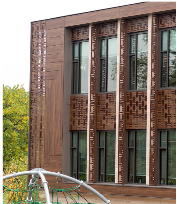
D.C. Bilingual Public Charter School | Product: Max Compact Exterior | Decor: Amazon #0922 NT | Photo Credit: PPSI | Architect: Hord Coplan Macht (HCM)
